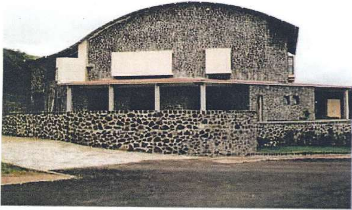
Geometric forms achieve their effect even when used with the local stone masonry.
