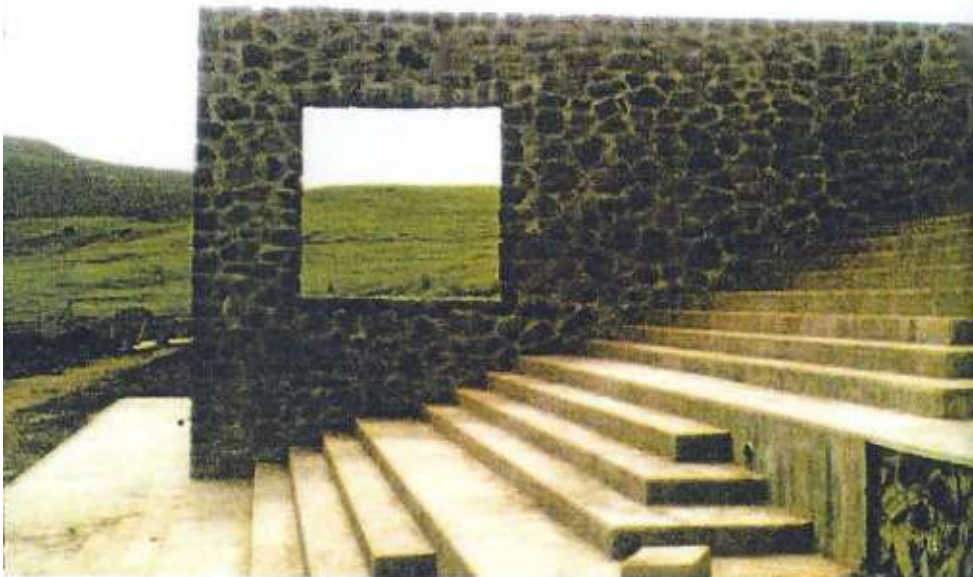
'wall feature at obstacle track'.
